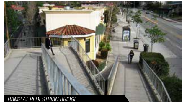
RAMP AT PEDESTRIAN BRIDGE
