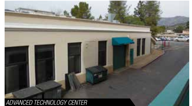
ADVANCED TECHNOLOGY CENTER
